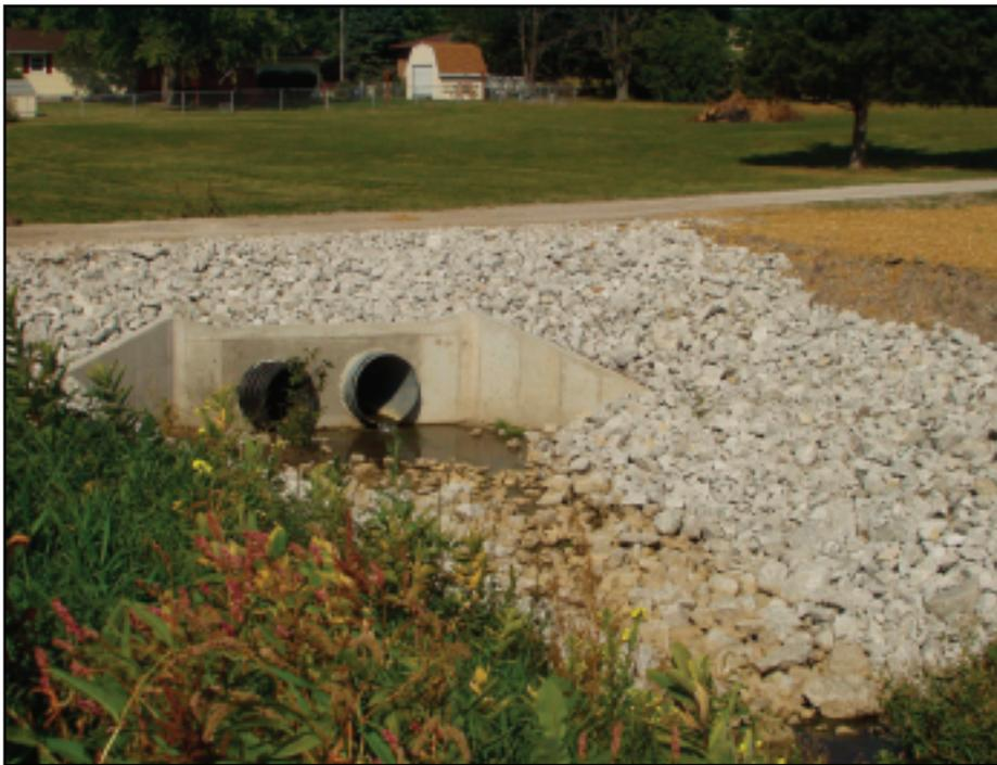
Outlet to newly installed storm drain from school, riprap around headwall and slopes.
