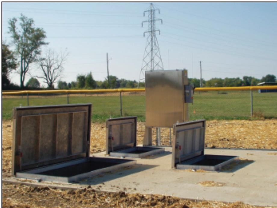
Open access to concrete septic tank. Control panel is in center background. Photo credits: Issy Weaver.
